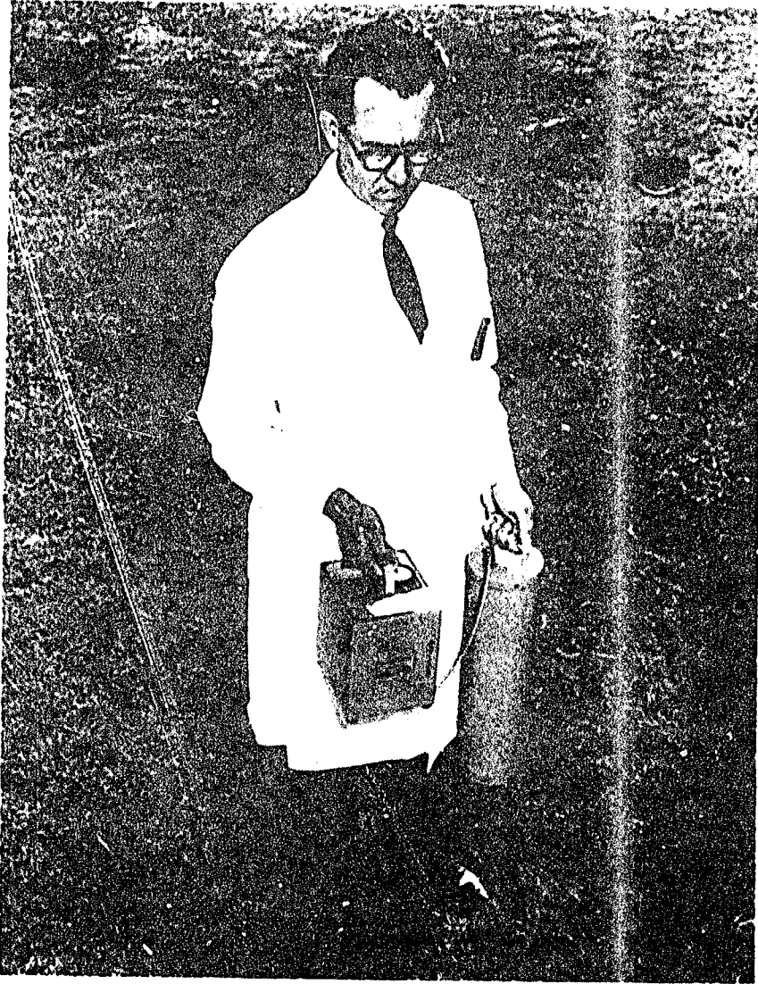
Figure 9 ^3_2\text{He} -FILLED NEUTRON COUNTER
